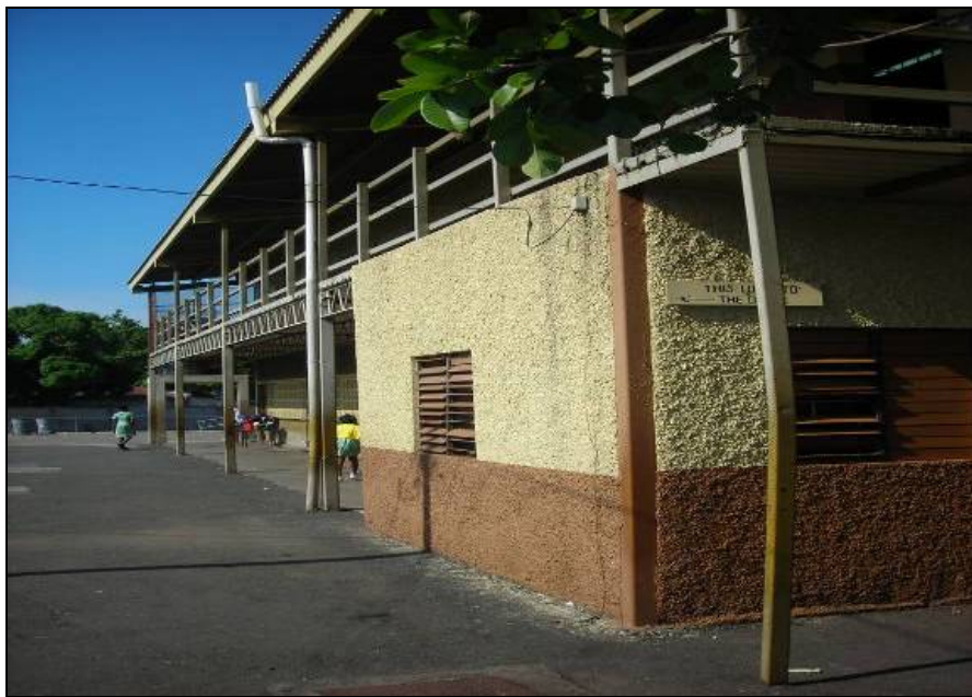
Figure 7. Grade 5 block (second floor) at St. Alphonso Primary School.
