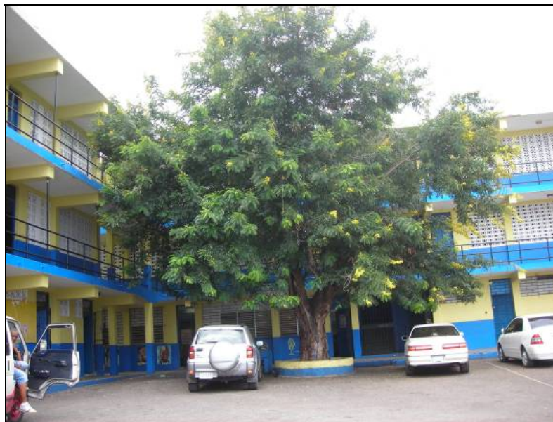
Figure 11. Inside Bedford Primary School. Grade 5 block on third floor (top left corner).
